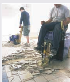
Removes the worst of today's glued down floors, including ceramic and wood
